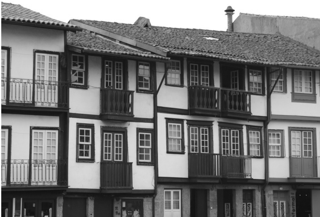
Buildings in the historic core of Guimarães. Photograph by Jorge Correia.
